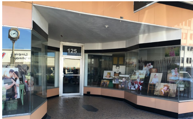
Above: Longview, Texas. Modernized historic storefront with recessed entry, aluminum display windows, and clad in structural glass. The tile entry also remains in place.
