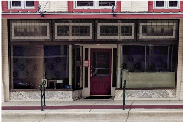
Above: La Grange, Texas. Copper storefront example (1900-1930s).
